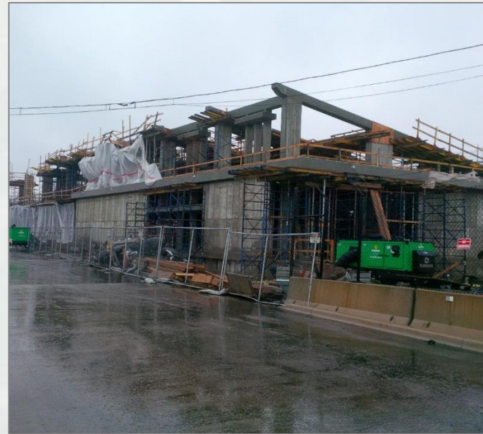
Building Construction as of 21 Dec 2015
