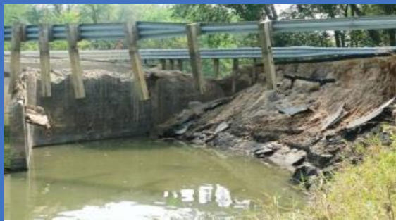
C. Roads & Bridges
