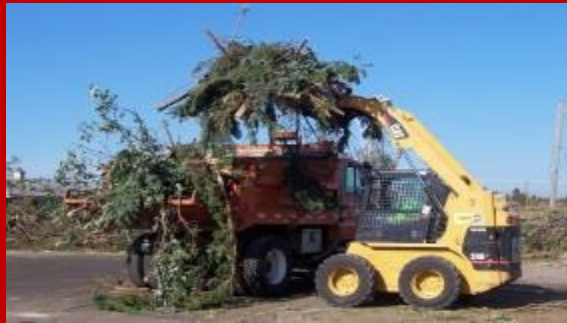
A. Debris Clearance
